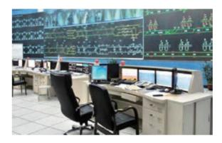
$\rightarrow$  The first Traffic Integrated Automation System(TIAS), was applied to China's first fully-automatic unmanned subway, Beijing Yan-Fang Line
