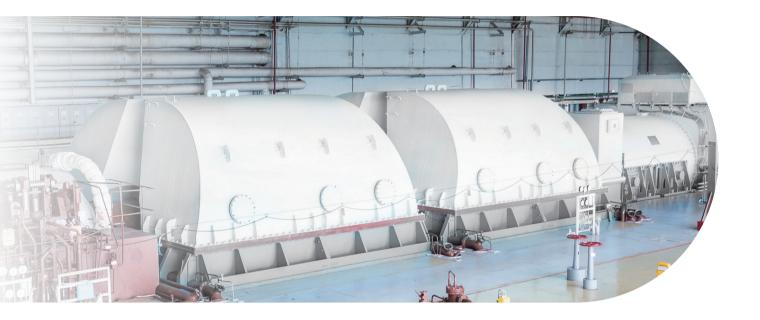
Developed the first-generation DEH, which was successfully put into operation in Jilin Changshan Power Plant Obtained the first DEH patent certificate, enabling the successful application of the DDV valve technology in DEH and breaking the constraints of electrohydraulic converters on DEH
